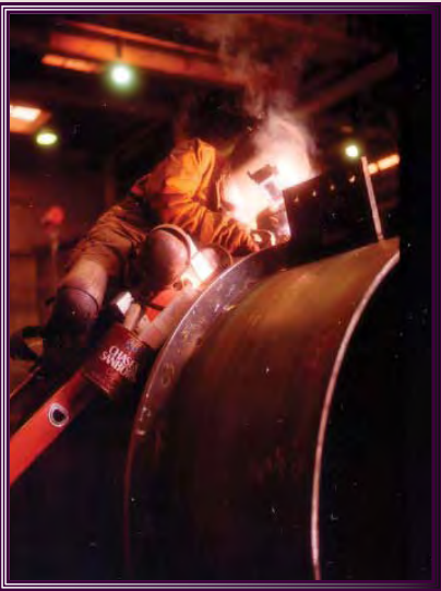
Pressure Vessel Fabrication - Seattle, WA.
